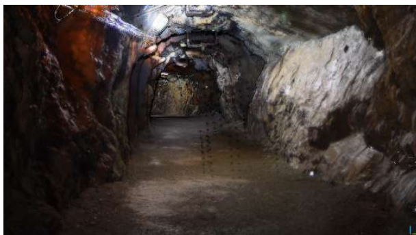
Figure 4. Render of a colored reference point cloud acquired with a survey-grade laser scanner
