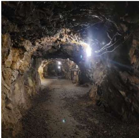
Fig. 2 Mapped locations: underground tunnel (aka adit)
