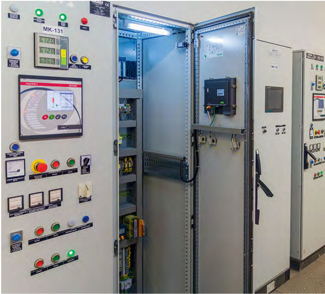
Figure 15: Switchboard with devices for controlling electrical network parameters as an example of binding the digital and physical assets [166]
