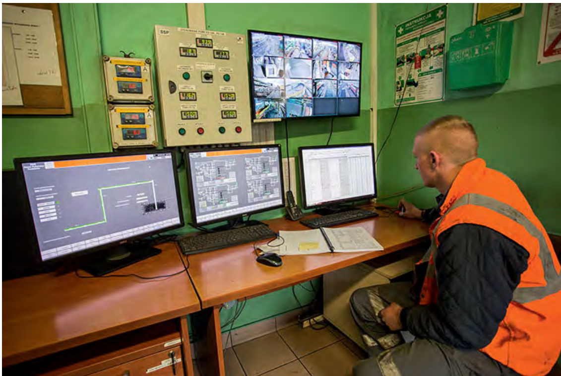
Figure 14: Control room of technological process with SCADA system at ZWR District [161]
