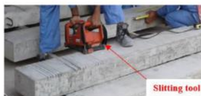
(a) Cutting groove with slitting tool.
