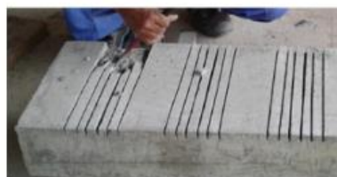
(b) Removal of concrete between the grooves.
