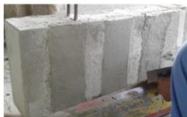
(d) Final layer of mortar and finishing of the surface (discontinuous configuration).
