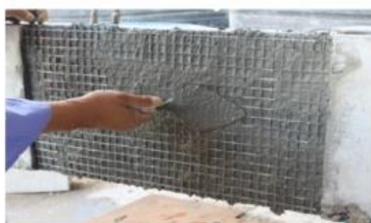
(c) Installation and full impregnation of first layer of fabric (continuous configuration).
