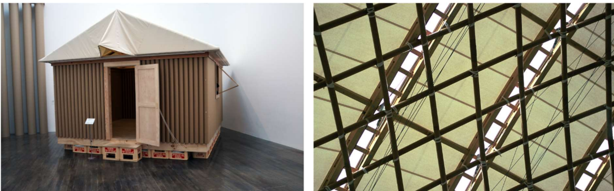
Figure 2.4. Examples of the architecture of Shigeru Ban with paper tubes; (a) Paper Log House; (b) Japan Museum 4 .
