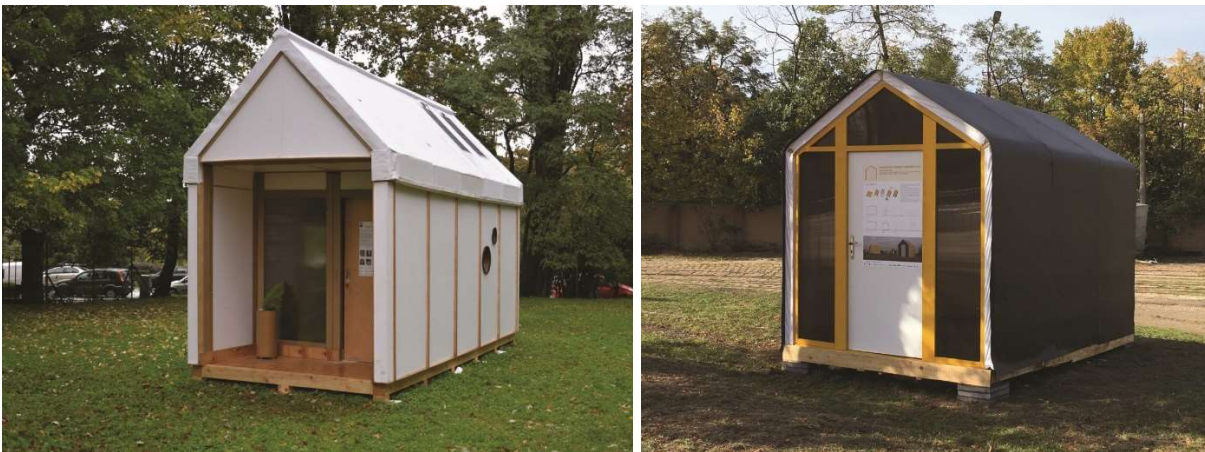
Figure 2.17. Paper-based buildings: (a) House of Cards prototype; (b) TECH 04 prototype 24 .
