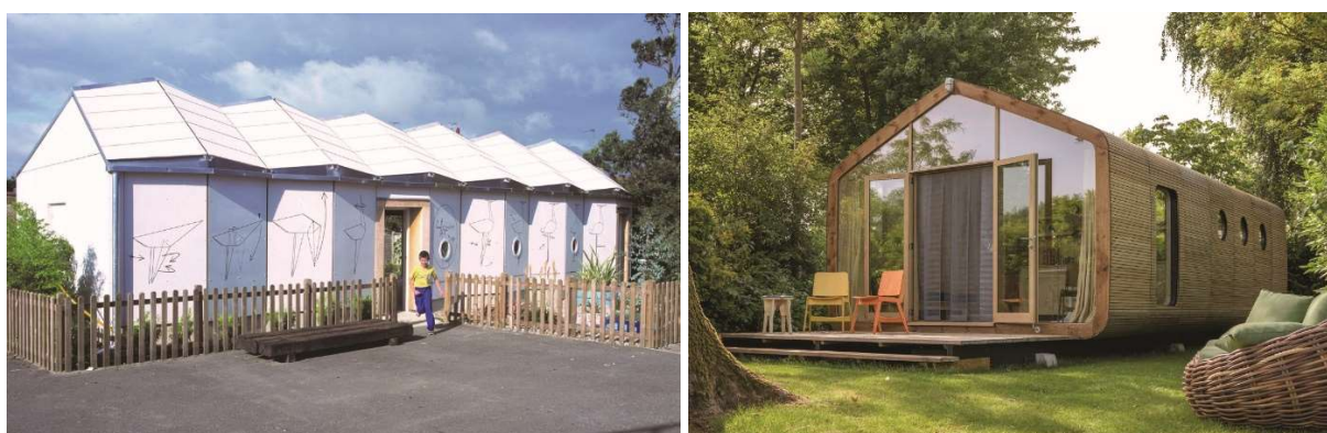
Figure 2.16. Paper-based buildings: (a) Westborough Primary School building; (b) Wikkelhouse 22 .
