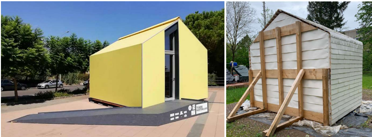
Figure 2.18. Paper-based buildings: (a) Archicart prototype; (b) Full Performance Paper House prototype 25 .
