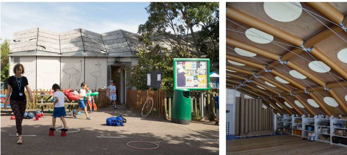
Figure 2.5. Examples of modern paper-based architecture; (a) Westborough Primary School; (b) Ban's studio at Kyoto University of Art and Design 5 .
