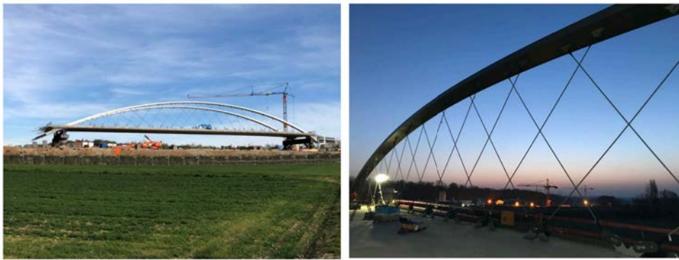
Figure 3.27 The NAB over Odra river made with CFRP hangers [63]
