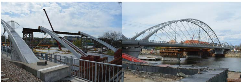
Figure 4.11 Photos of NAB in Cracow [12]
