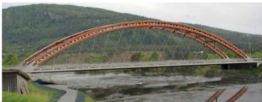
Figure 3.22 The Steien bridge [154], the first network arch bridge made of timber [72]
