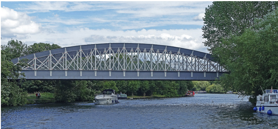
Figure 3.3 The Windsor Railway tied-arch bridge [159]
