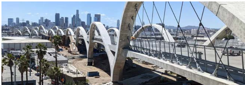
Figure 3.21 Illustrations of inclined (a), (b) inwards and (c) outwards network arch bridges
