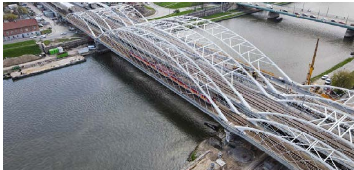
Figure 3.18 Illustrations of network arch bridge with HD arch section [146]
